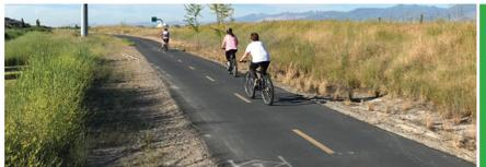
**Shared Use Paths** are paved paths/trails, typically 8-12' wide, constructed of asphalt or concrete, that accommodate pedestrians and bicyclists off street.
